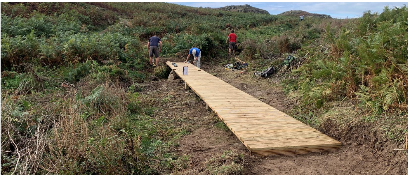
11 The new boardwalk at South Stream – L. Newman
